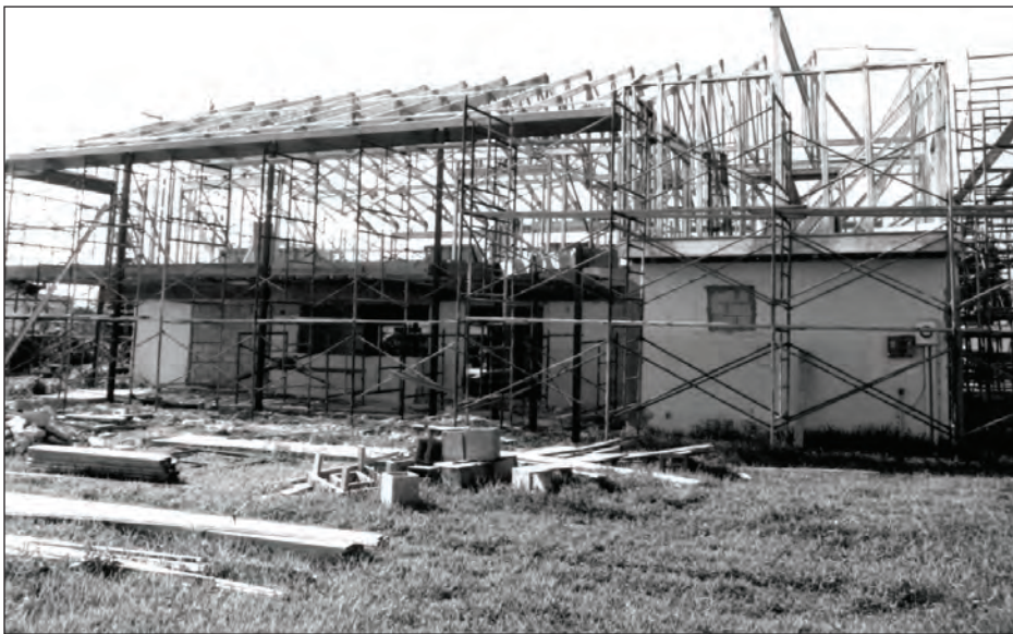
Figure 3-6. The owner of this flood-prone home in south Florida decided to build a new wood-framed second story on top of his masonry first story. The new second story is well above the BFE.
