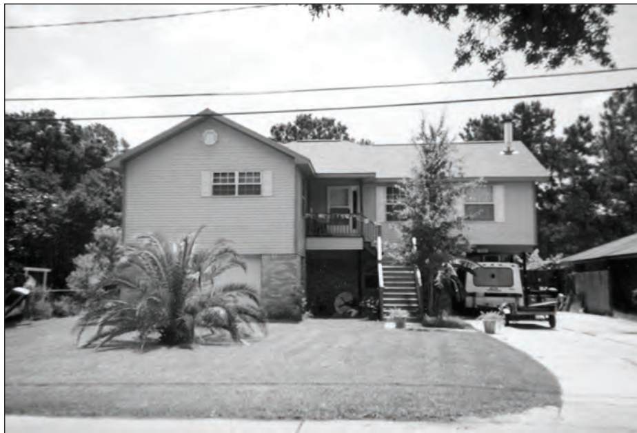
Figure 3-4. Retrofitted home elevated on extended continuous foundation walls.
