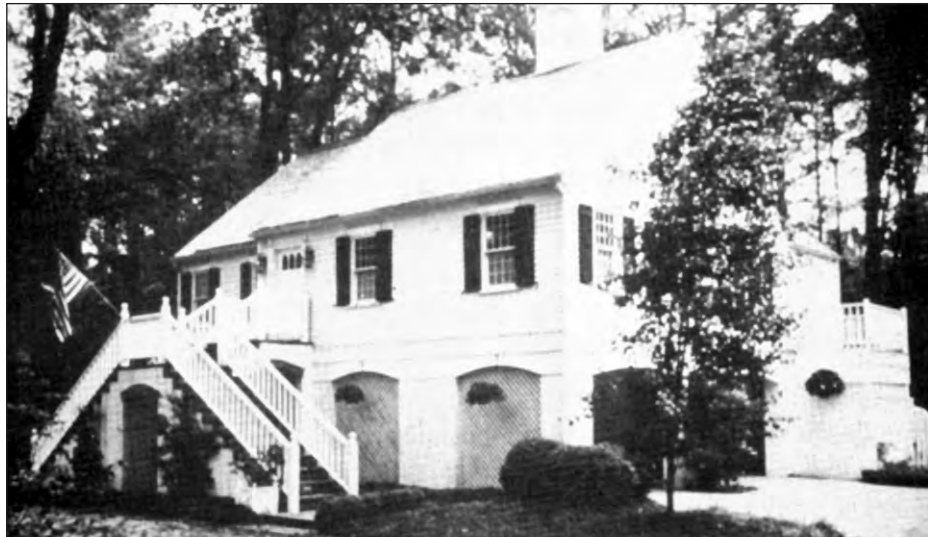
Figure 2-2. The home was elevated in a way that added to both its appearance and its value.
