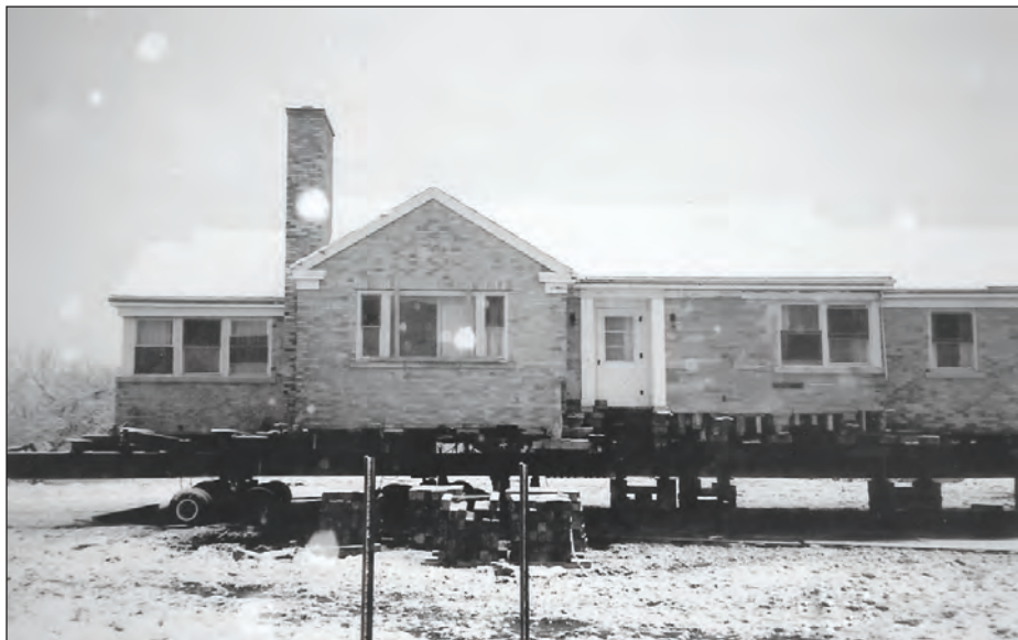
Figure 7-3. The move to the new site begins.
