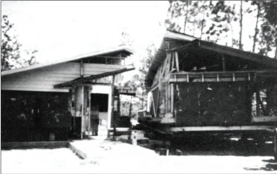
Figure 7-1. When a home is too large to be moved in one piece, it may have to be cut into sections that can be moved separately and then reassembled at the new site.
