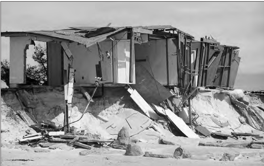
Figure 2-5. The extreme impact of large, fast-moving waves, combined with the removal of supporting soil by erosion and scour, can have devastating effects on buildings exposed to coastal flooding. This home along the Gulf of Mexico shoreline was destroyed during Hurricane Opal.
