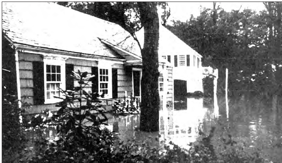
Figure 2-3. Now the home (in the background) is protected from flooding, unlike the flooded home in the foreground.
