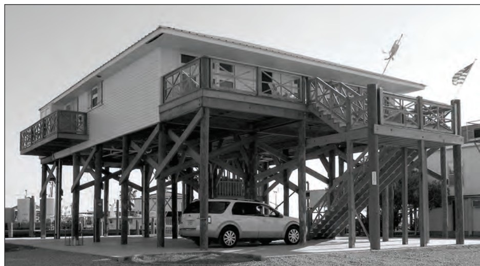
Figure 3-5. This coastal home was elevated on piles so that it is less vulnerable to damage from coastal flooding.
