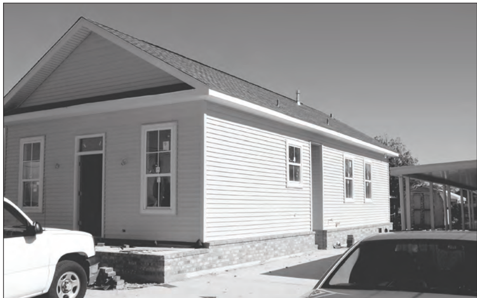
Figure 7-21. Typical mitigation reconstruction project.
