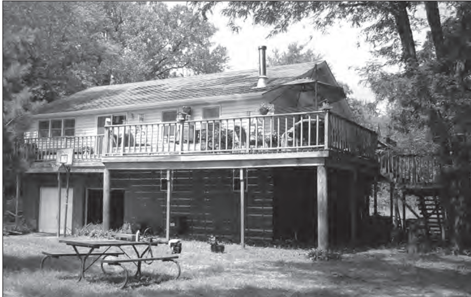
Figure 5-2. This home in Cedar Falls, Iowa, was elevated one full story. The garage and storage area are at the home's original elevation.
