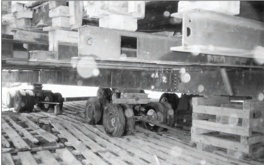
Figure 7-2. Trailer wheel sets are placed beneath the lifting beams.
