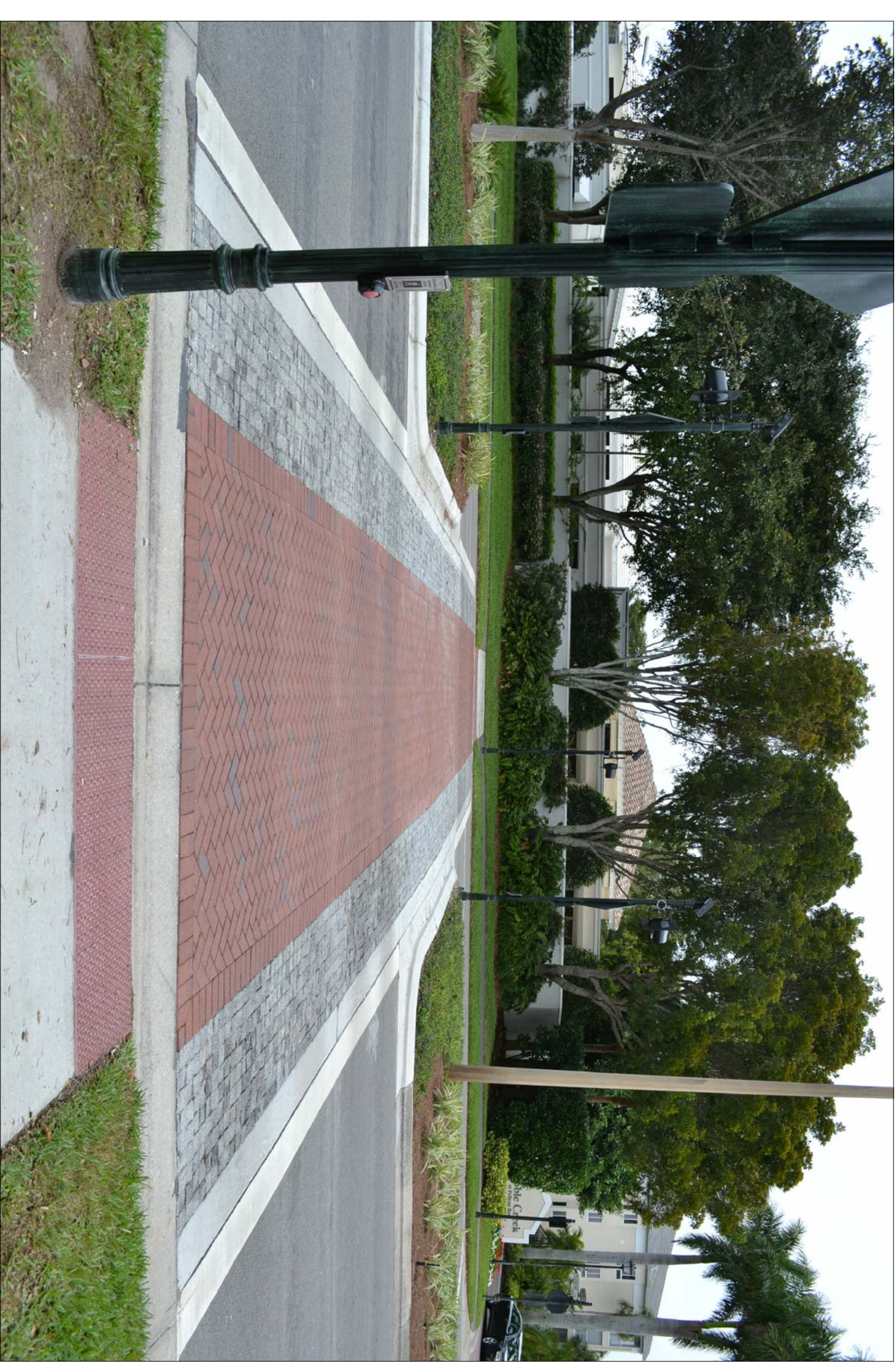
PAVER CROSSWALK WITH COBBLE BANDS
