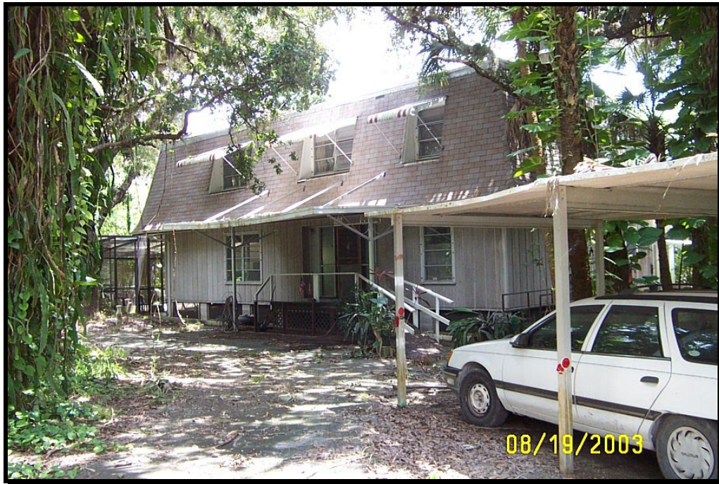
Photo 4. Main residential dwelling (Mobile home with additions and roof covering entire pieced together structure).
