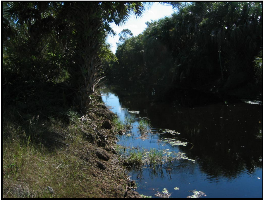
Photo 6. Canal at southern boundary
