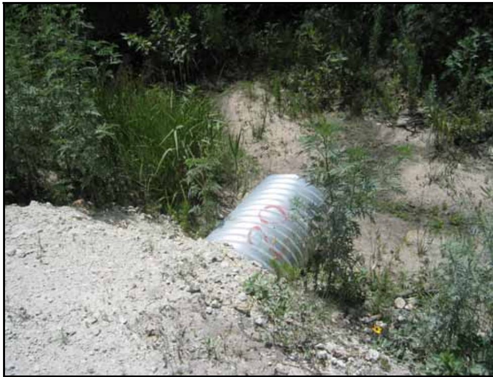
Photo 8. Lone culvert observed under 39 th Ave NE
