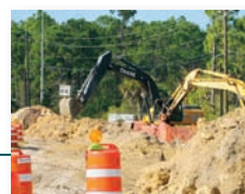
Intersection improvements are underway at Collier and Davis Boulevards.
