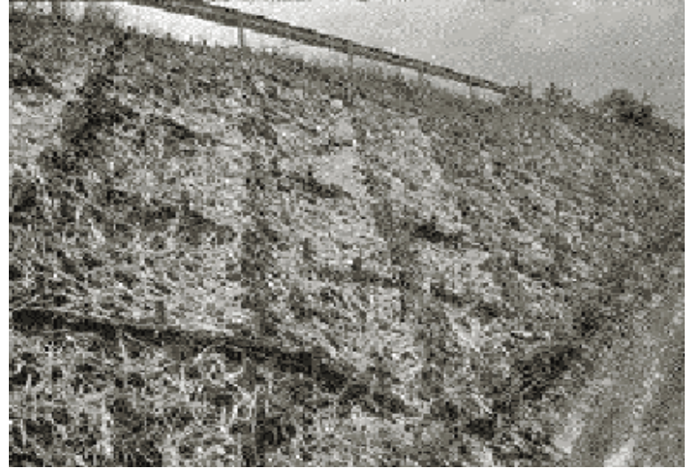
Figure 5-1. Erosion control mattings
