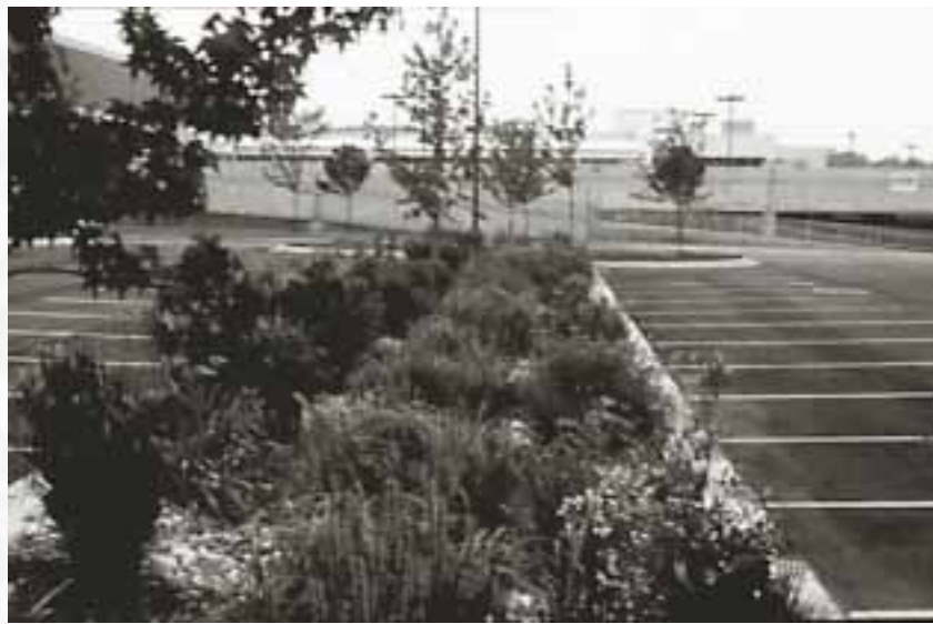
Figure 1-1. Parking lot bioretention area
