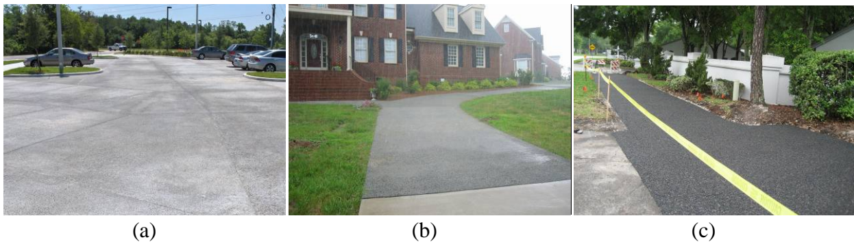
Figure 3.2-3 Examples of Pervious Pavement (a: Parking Lot, b: Driveway, c: Walking Path)
