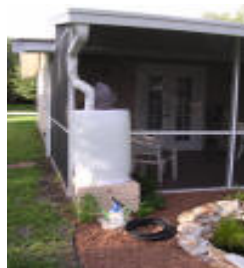
Figure 3.5-1 Rainwater Harvesting with a Rain Barrel
