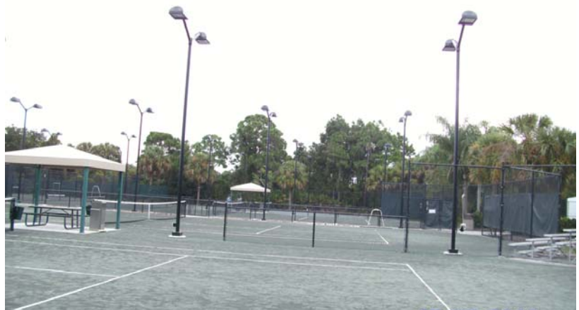
Lighting Project Completed at Pelican Bay CP Tennis Center
