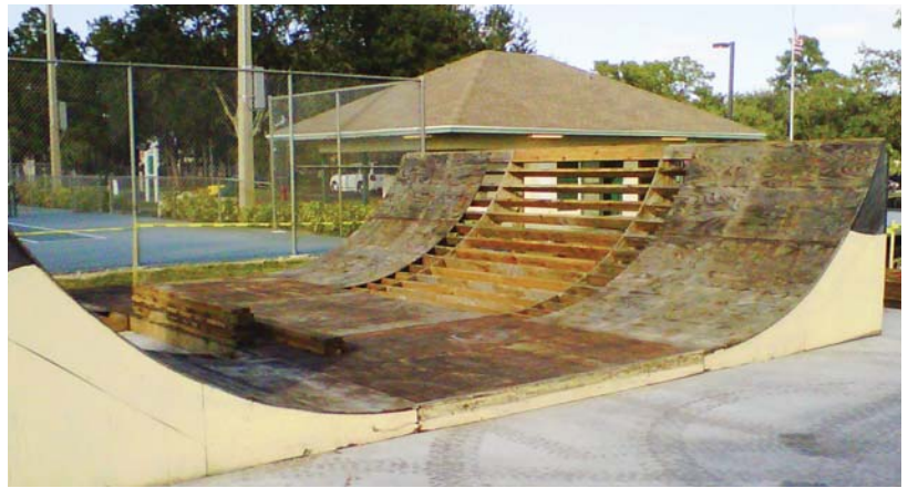
Construction at Immokalee Sports Complex - skate ramps
