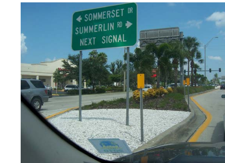
COLONIAL BLVD (CR884), LEE COUNTY CRUSHED SHELL USED AT NOSES OF MEDIANS FROM CLEVELAND AVE TO MIDPOINT BRIDGE
