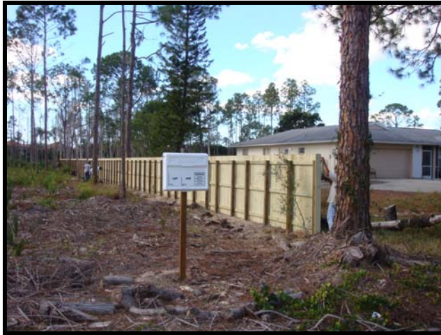
Six-foot high, wood privacy fence along the eastern half of the northern boundary of the Logan Woods Preserve. Photo by Christal Segura
