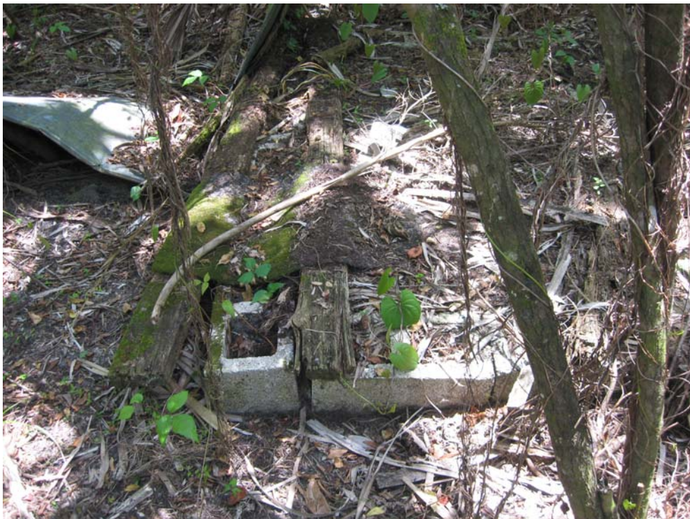
View of apparent septic system adjacent to former wooden structure
