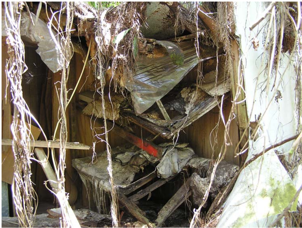
View of interior of trailer – west side (southwest portion of property)
