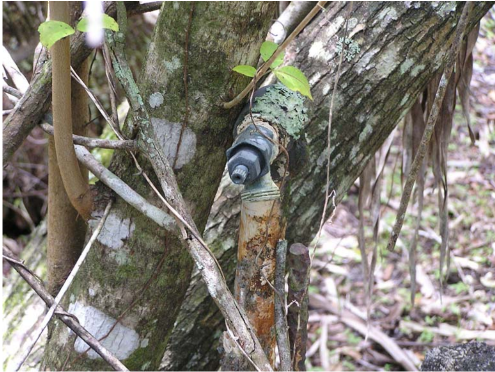
Water pipe and fitting adjacent to former wooden structure
