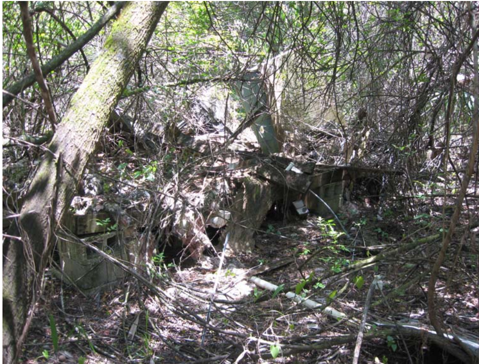
View of former wooden structure from north
