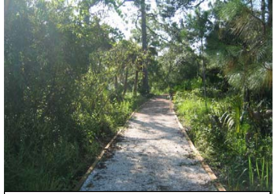
Trail section made of compacted limestone shell
