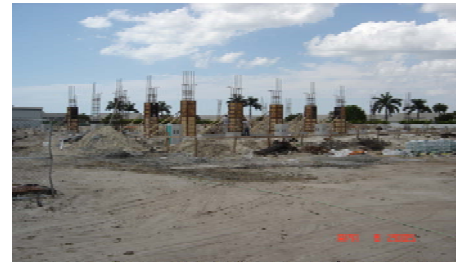
North Naples Government Services Center construction
