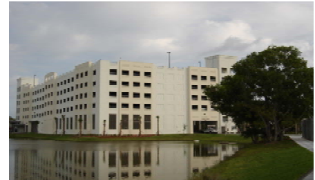
Campus Parking Garage
