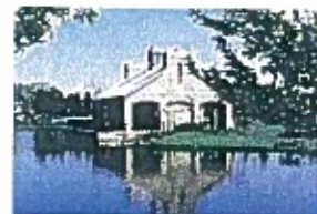
Shelter house at Homestead Park.
