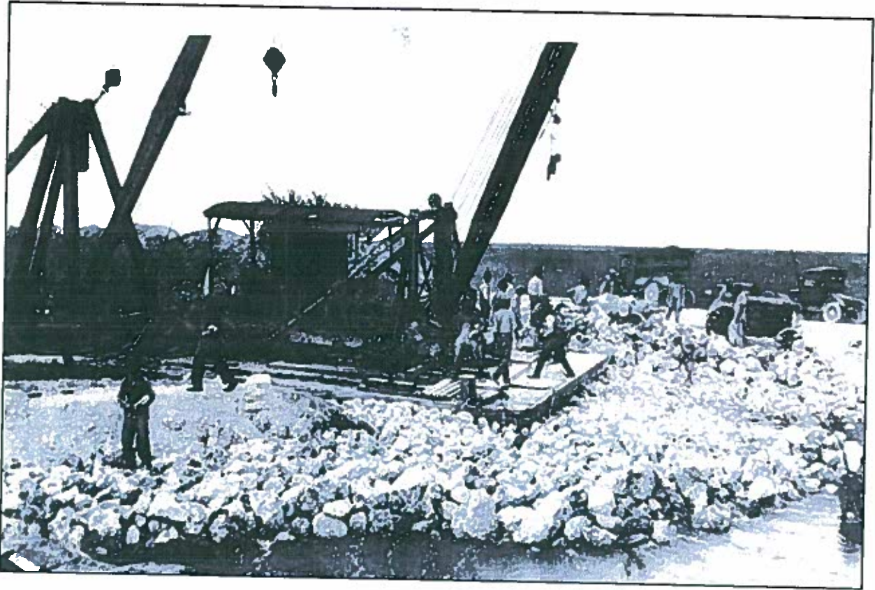
This picture from 1920 shows the men and machinery starting the Tamiami Trail, on the outskirts of Miami.
