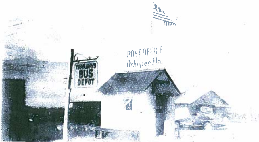
Ochopee Post Office, Gas Station and Garage, 1958
