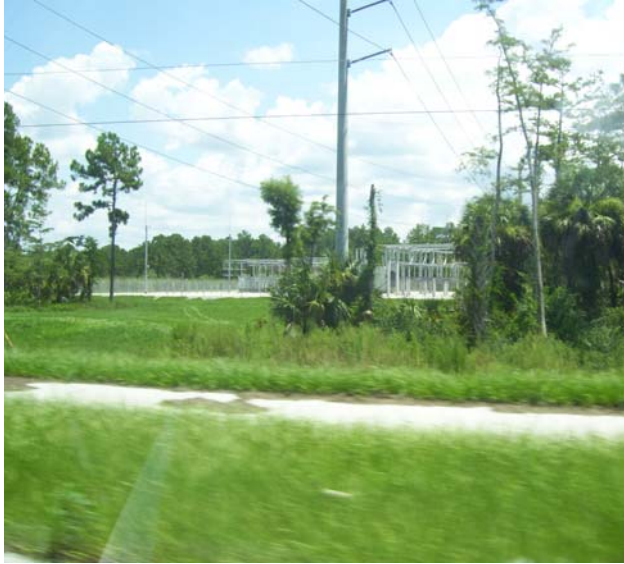
Orangetree Substation, Collier County
