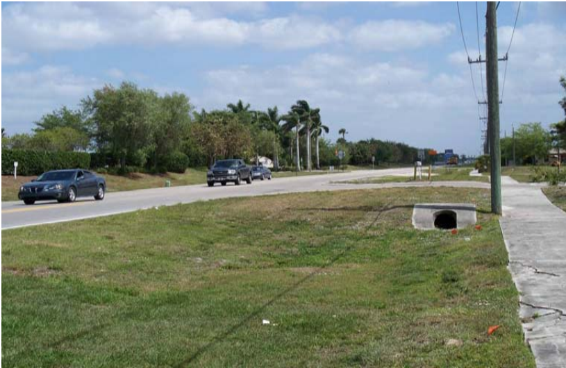
Sidewalk and Drainage along Oil Well Road
