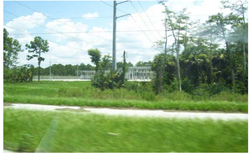
Orangetree Substation with Concrete Path
