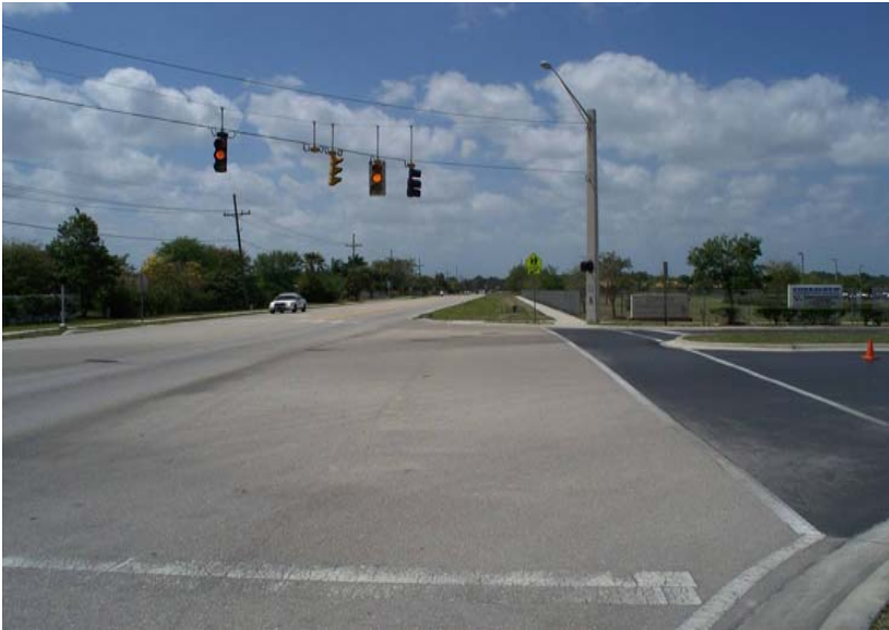
Intersection of Oil Well Road and Corkscrew Elementary School Entrance
