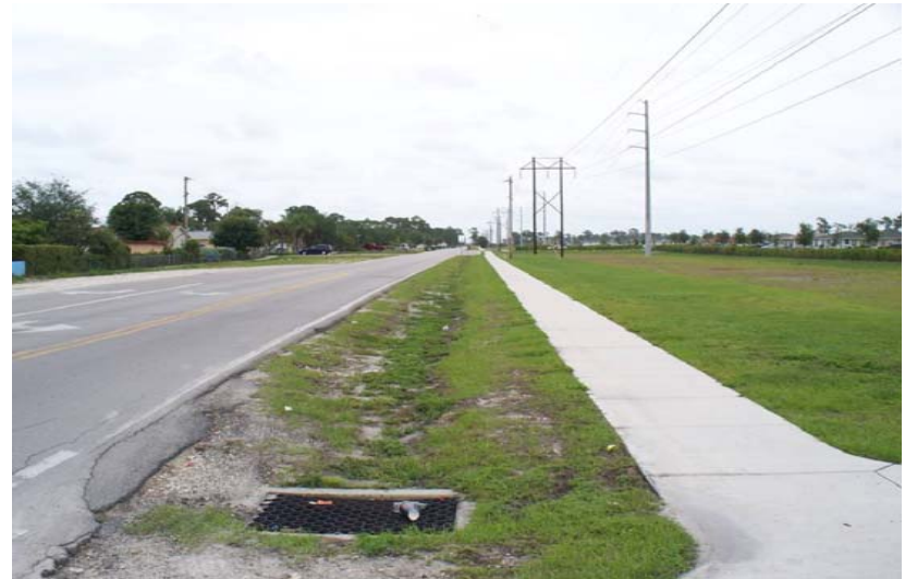
Drainage Feature, Sidewalk and FPL Easement along Little League Road
