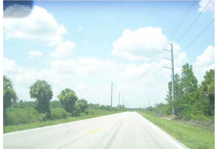
FPL Easement Road Crossing – Immokalee Road
