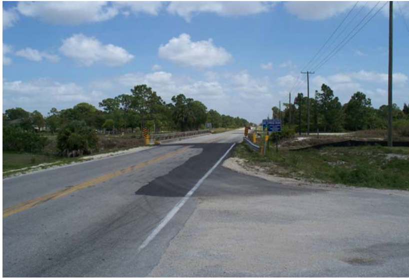
Oil Well Road – Golden Gate Canal Crossing
