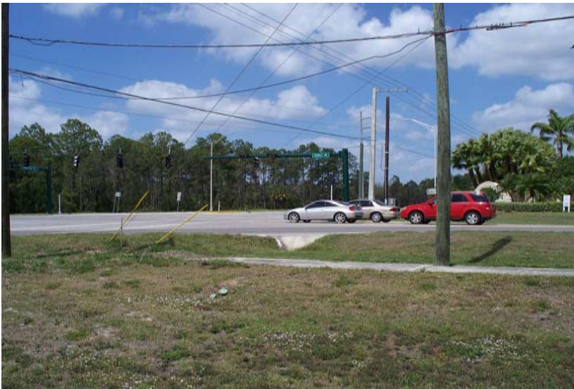
Sidewalk and Drainage at the Intersection of Oil Well Road and Immokalee Road
