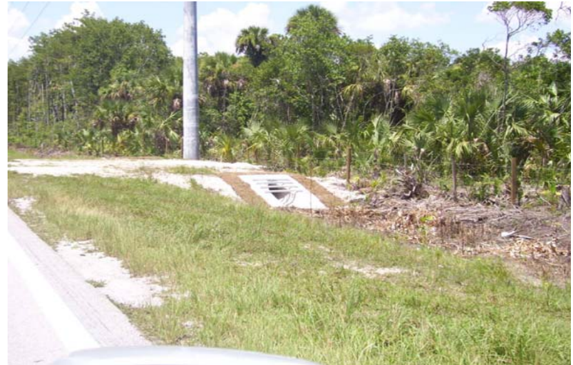
Drainage Structure along FPL Easement – Immokalee Road
