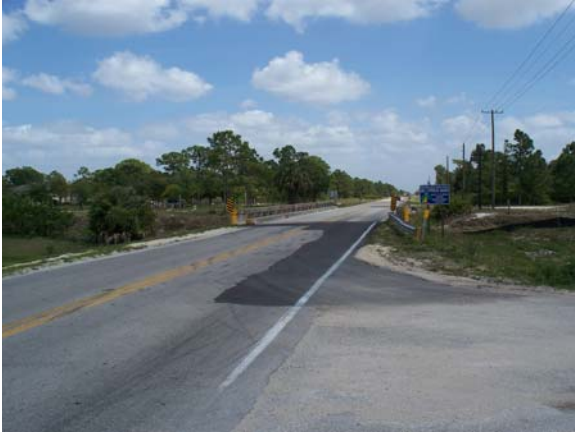
Golden Gate Canal Crossing – Oil Well Road
