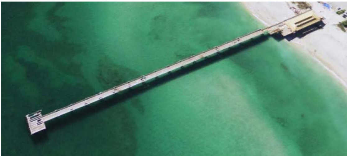
Photograph 3: Dania Pier was originally built over hardbottom. The pier includes a terminal section and a landward facility built on the deck.
