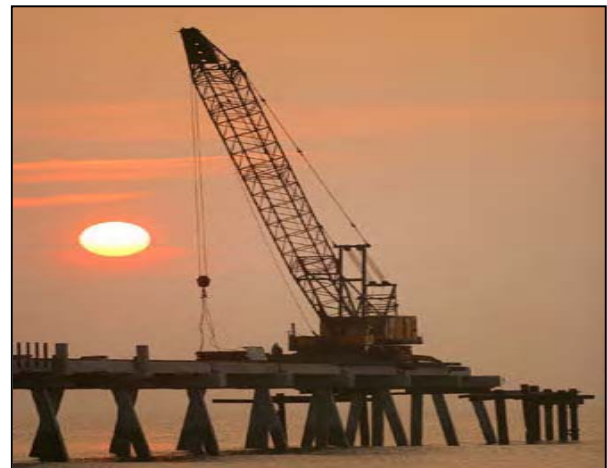
New Jacksonville Pier during construction
