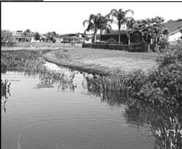
▲ Planted littoral zone in residential stormwater pond.
