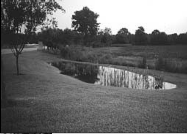
Pretreatment Sediment Basin ▲
