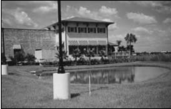
Man-made Stormwater Pond ►
