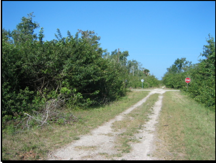
Photo 3: Looking west along 40 th Ave SE, from just east of Desoto Blvd. Gore parcels across Desoto on right and left. Road condition is rough.
