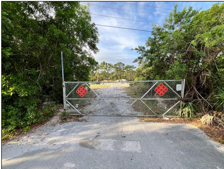
View to the south from Business Lane. (Photo Taken April 28, 2024)
