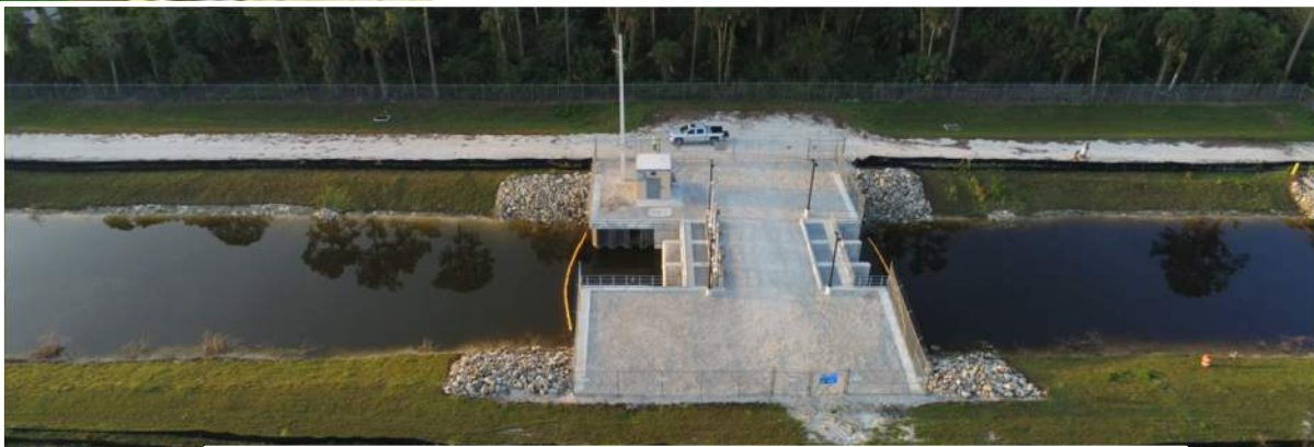
New Cypress Water Control Structure
