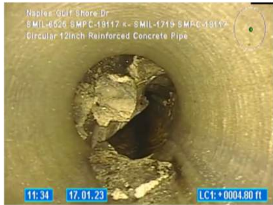
Collapsed Pipe
