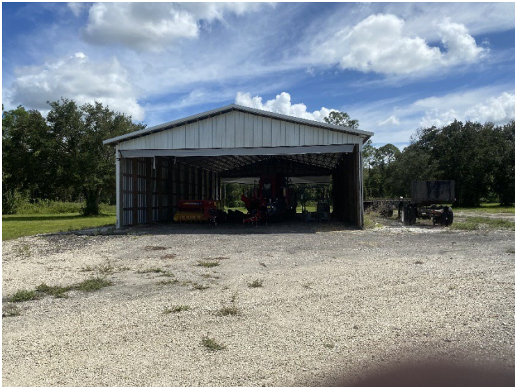
Large storage building
