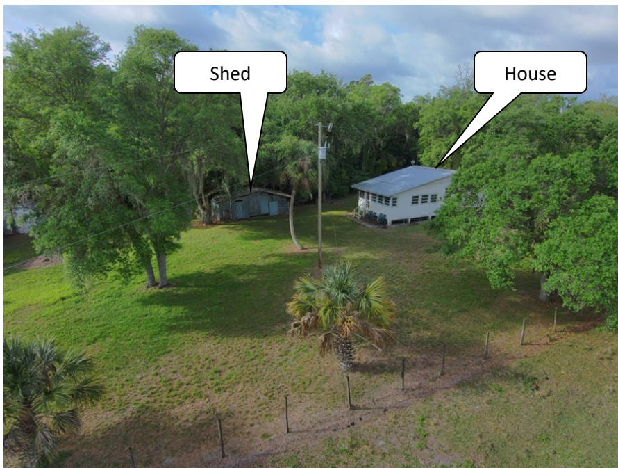
Figure 17 – Aerial views of Santamaria structures
