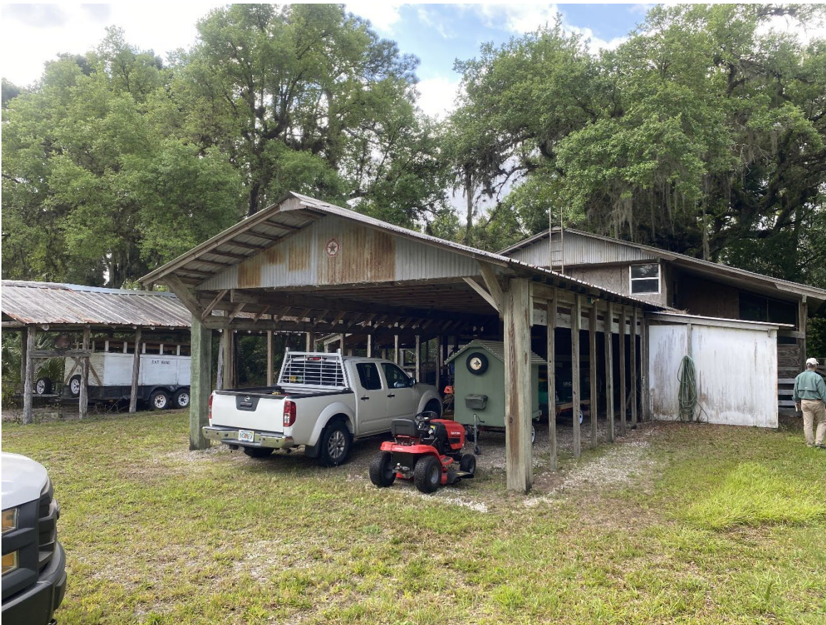
Pole barn with adjoining screened in area
