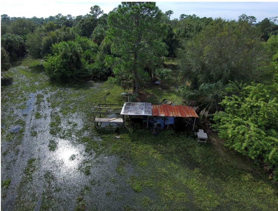
Figure 22 – Small, primitive pole barn
