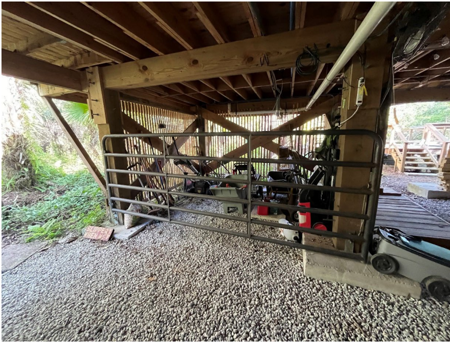
Gore Nature Center under house locked storage
