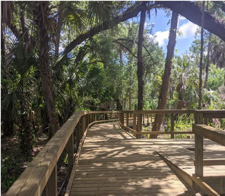
Gore Nature Center elevated boardwalk near buildings
