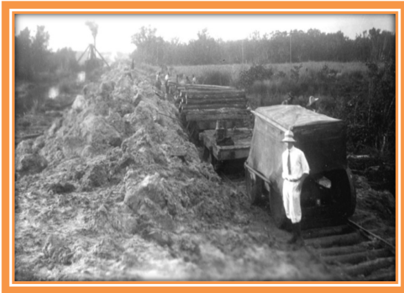
Construction site at the Tamiami Trail. Temporary railroad with Ford motor-car
