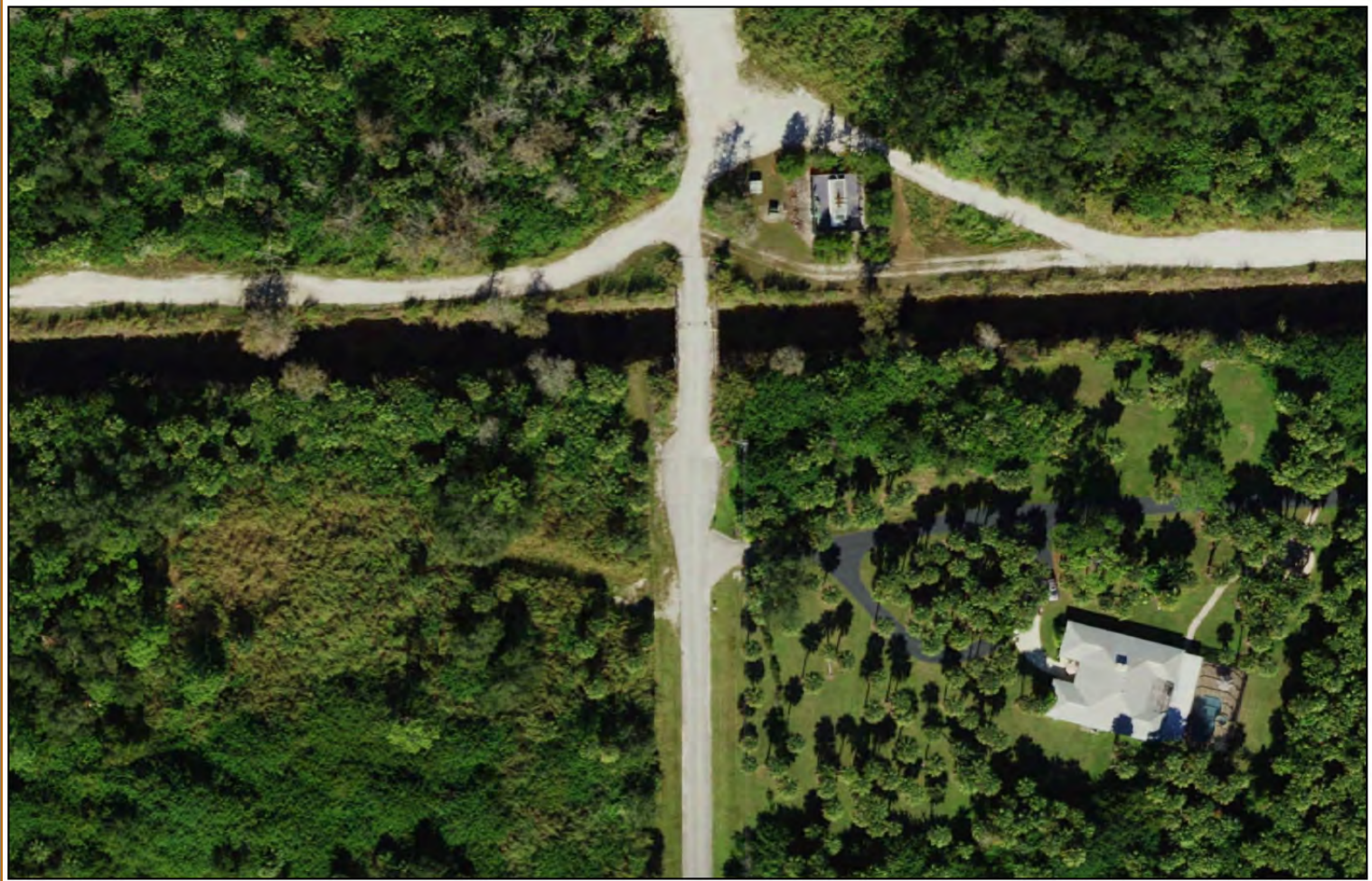
Location of Bridge #8: Existing Condition
