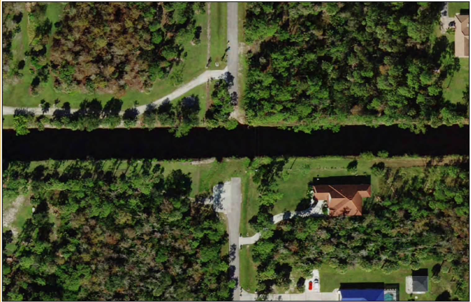
Location of Bridge #5: Existing Condition
