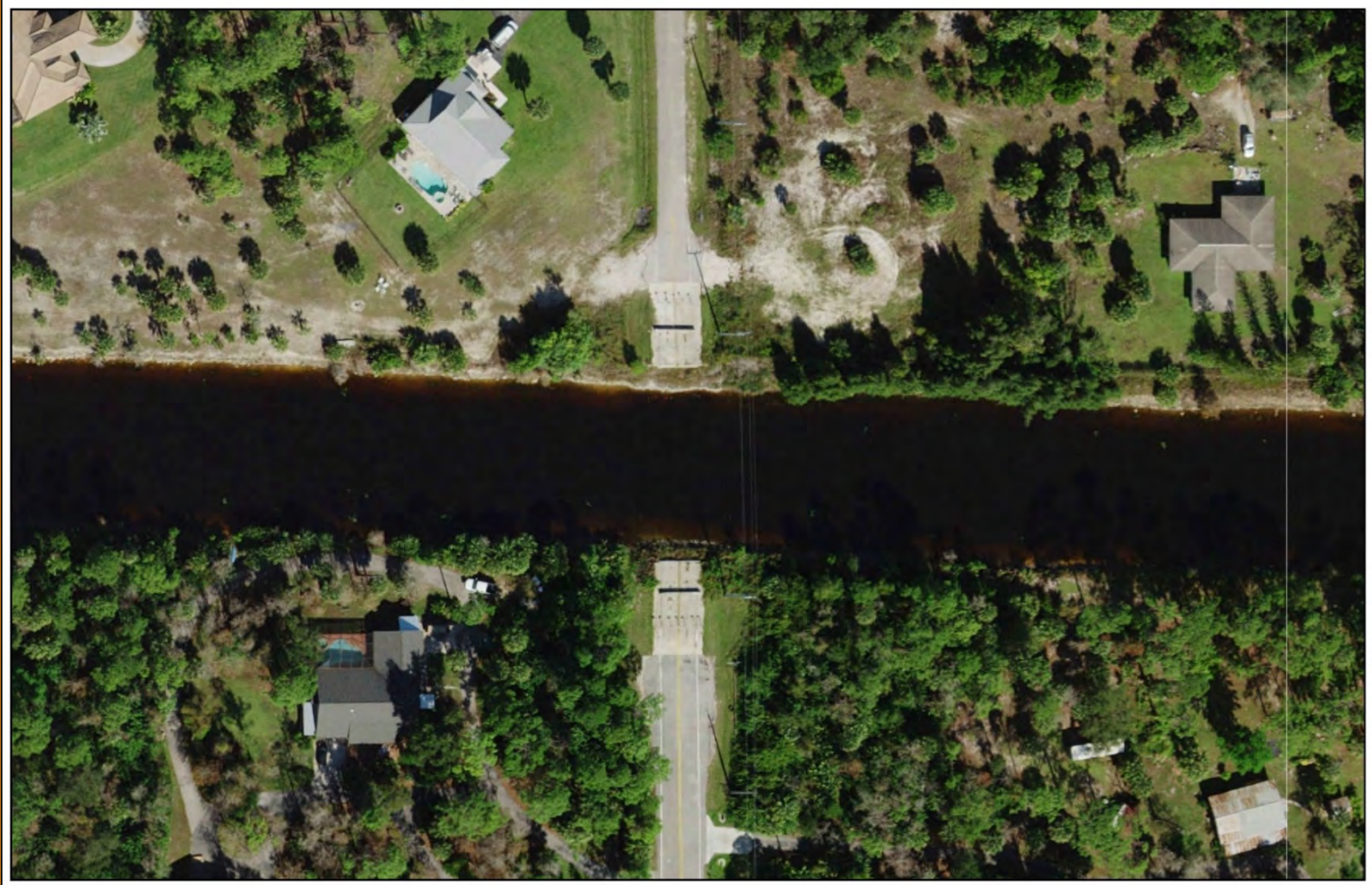
Location of Bridge #1: Existing Condition
