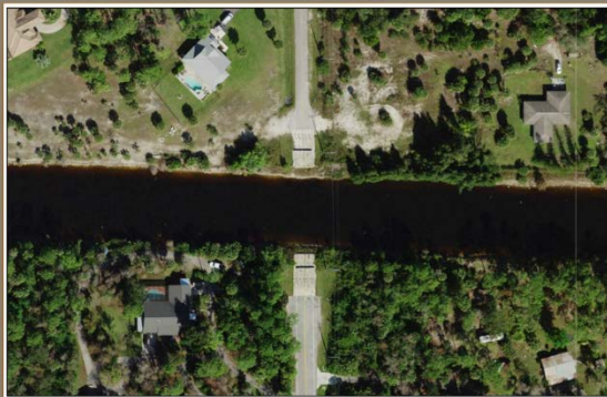
Location of Bridge #1: Existing Condition
