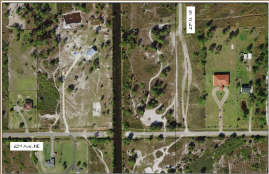
Location of Bridge #12: Existing Condition
