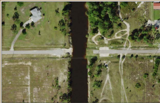
Location of Bridge #4: Existing Condition
