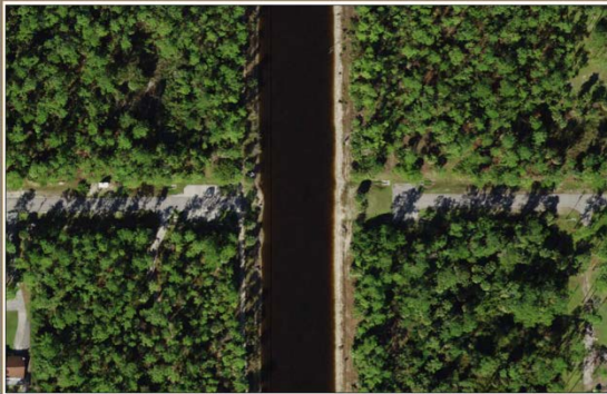
Location of Bridge #11: Existing Condition
