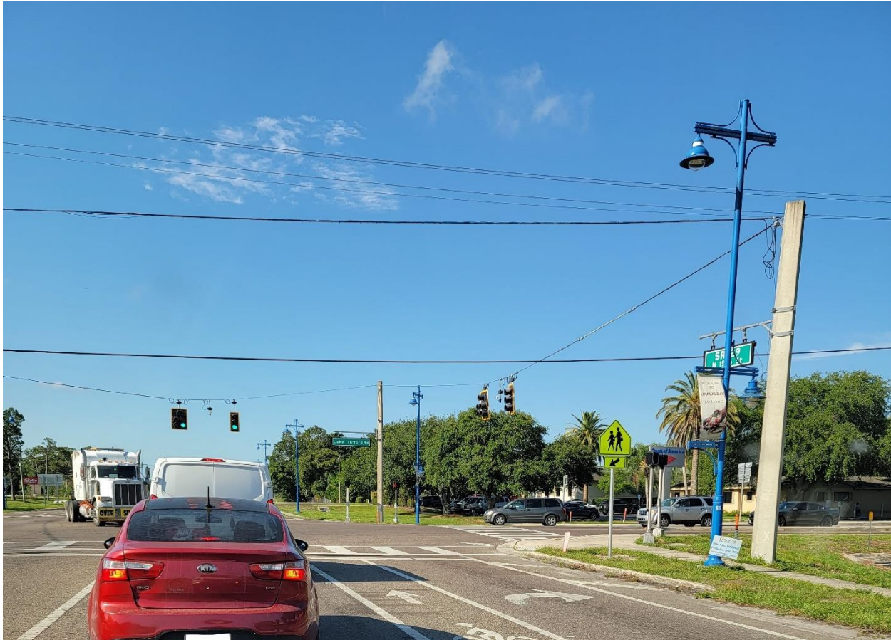
Figure 12. Unbuffered Bicycle facility found at the intersection of SR 29 and Lake Trafford Road
