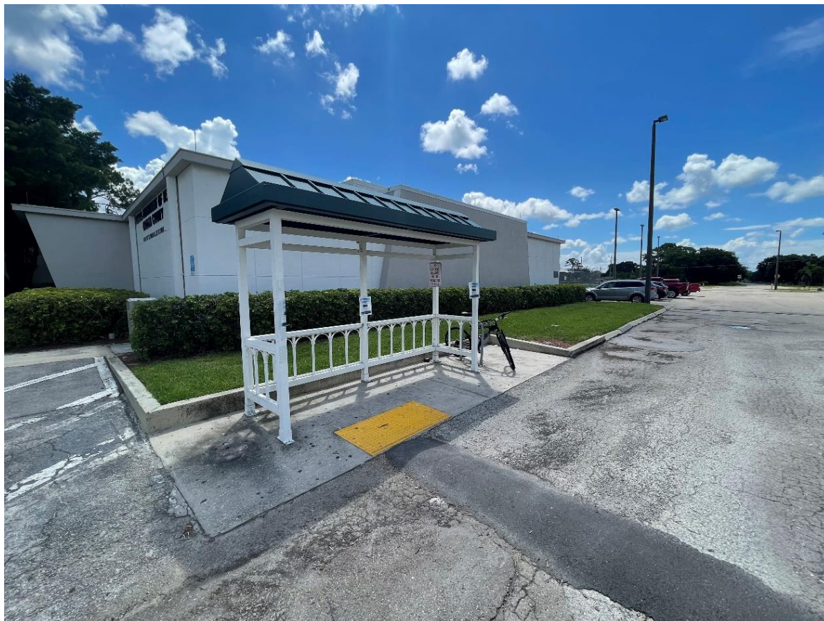
Figure 14. Existing Transfer Facility
