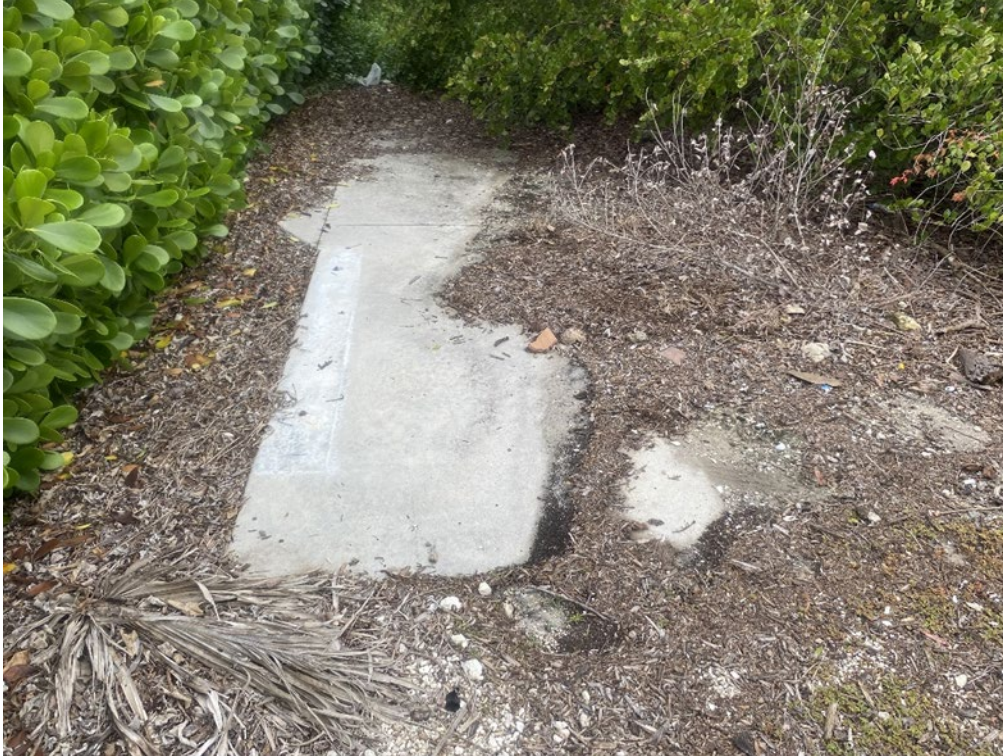
Visible portion of 16'x16' cement slab on north side
