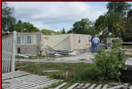
Roof & walls collapsed, Single Family (SF)
