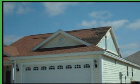
Few missing shingles, covered, no impending weather
