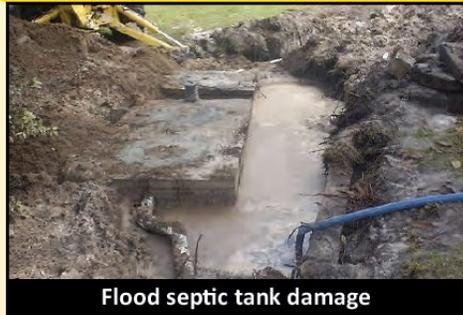
Flood septic tank damage
