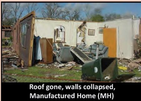
Roof gone, walls collapsed, Manufactured Home (MH)
