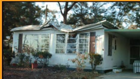
Roof partially collapsed, Manufactured Home (MH)
