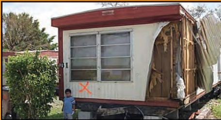
Wall coverings damaged and exposed, Manufactured Home (MH)
