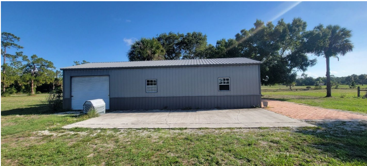
Figure 20 - Storage Building south of pond
