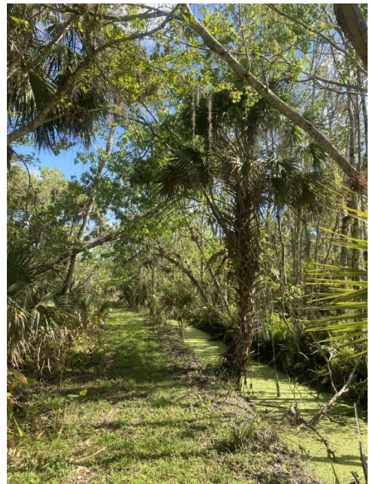
Ditch along southern boundary
