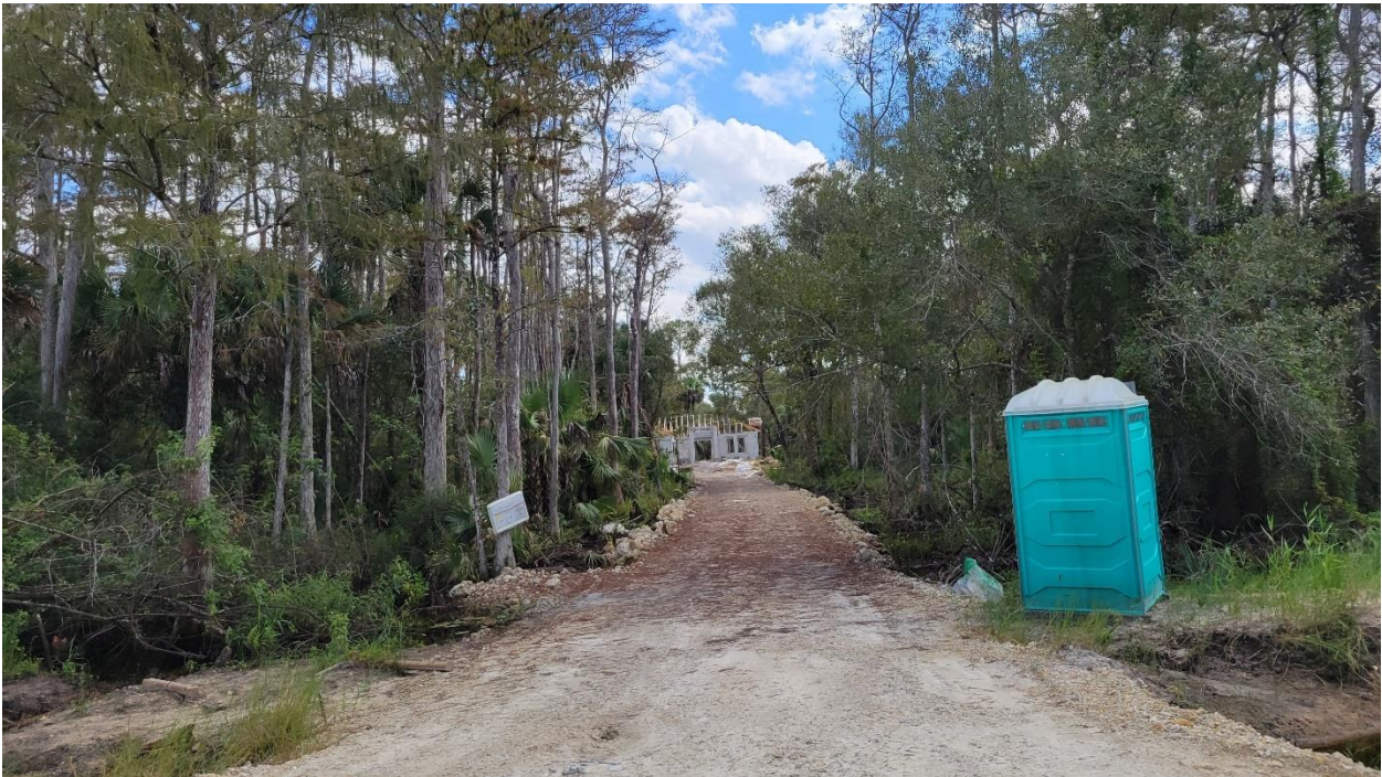
Construction within Horsepen Strand
