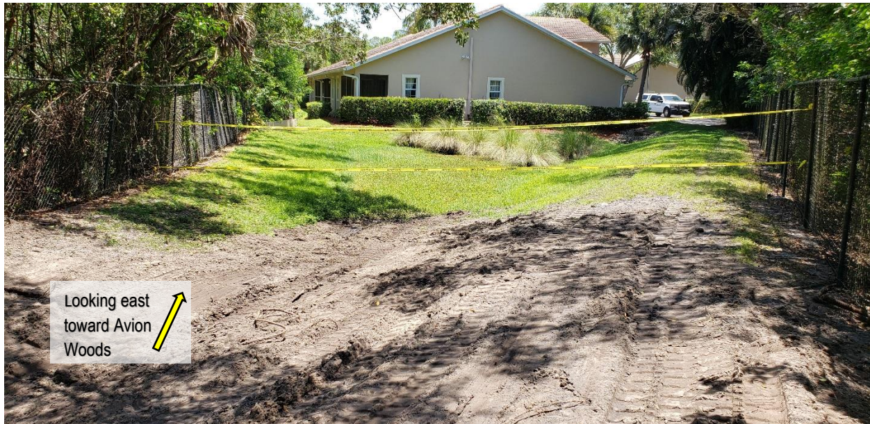
Figure 13. Sewage line repair at Avion Woods stormwater retention area May 6, 2022.
