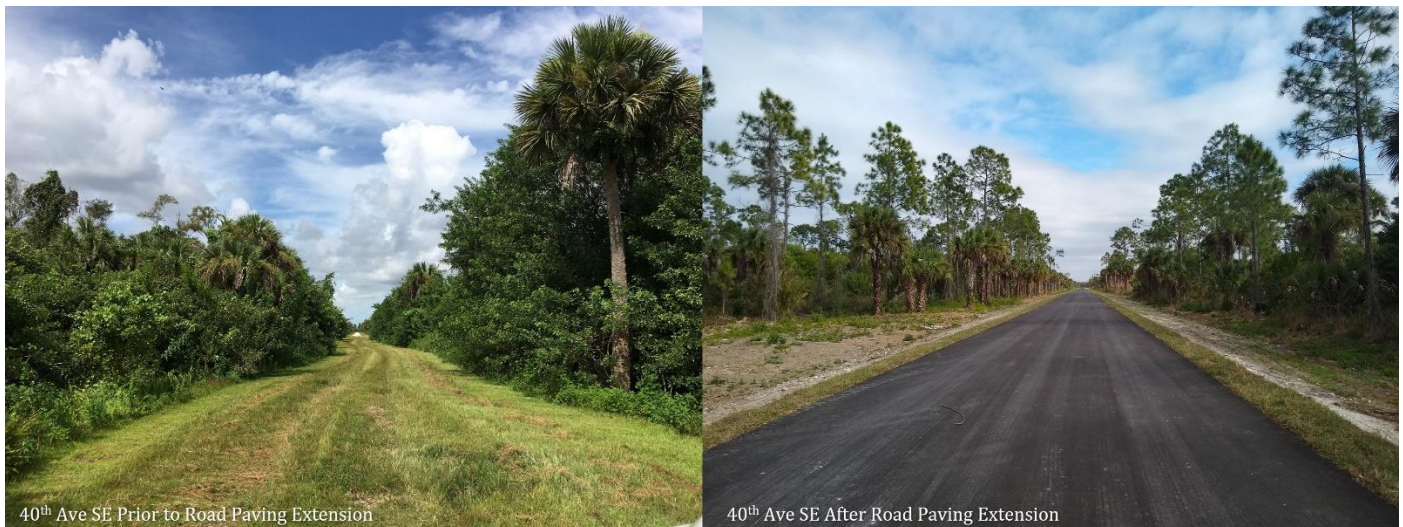
Photo 14. View of the access to 40 th Ave SE prior to paving the road and current conditions.
