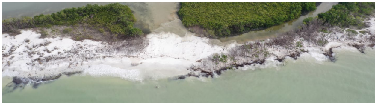
Park shoreline where the eroding beach is further impacted by Hurricane Ian
