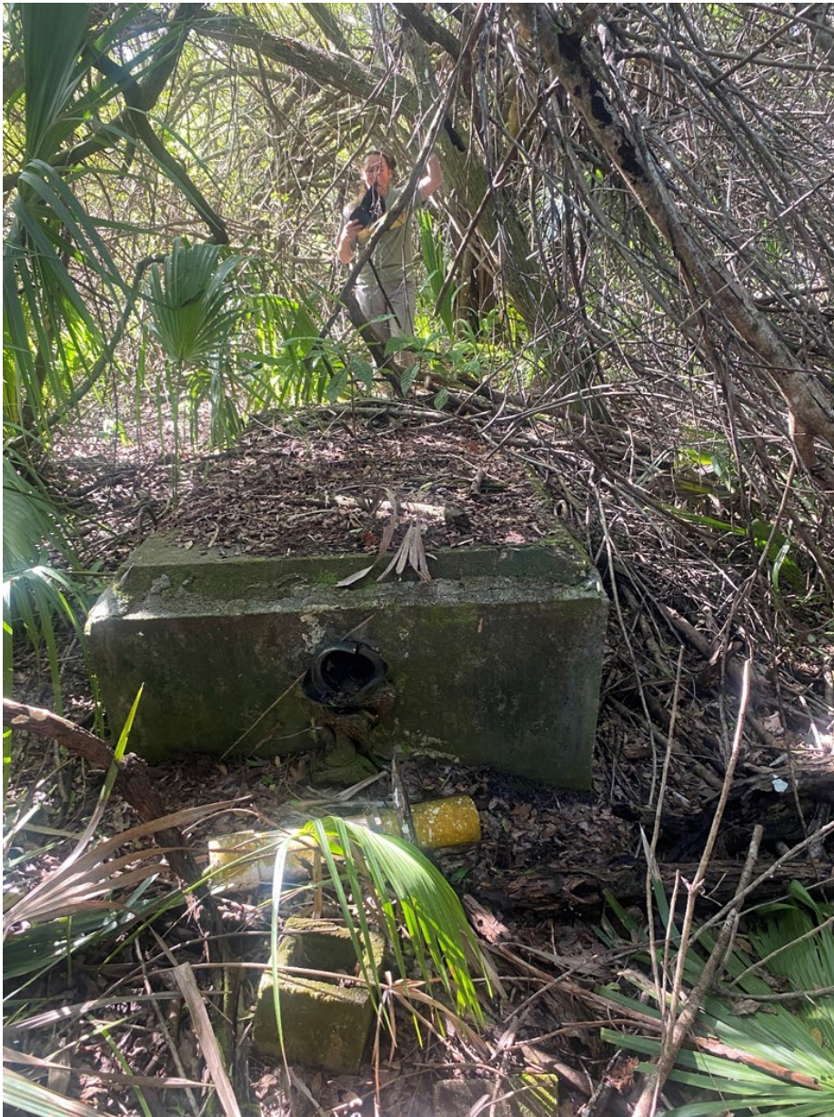
Figure 20 - Old Septic Tank
