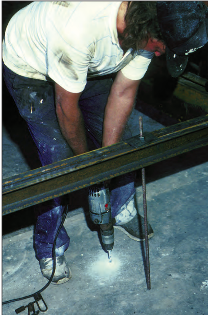
Figure 77 ... install anchors ...
