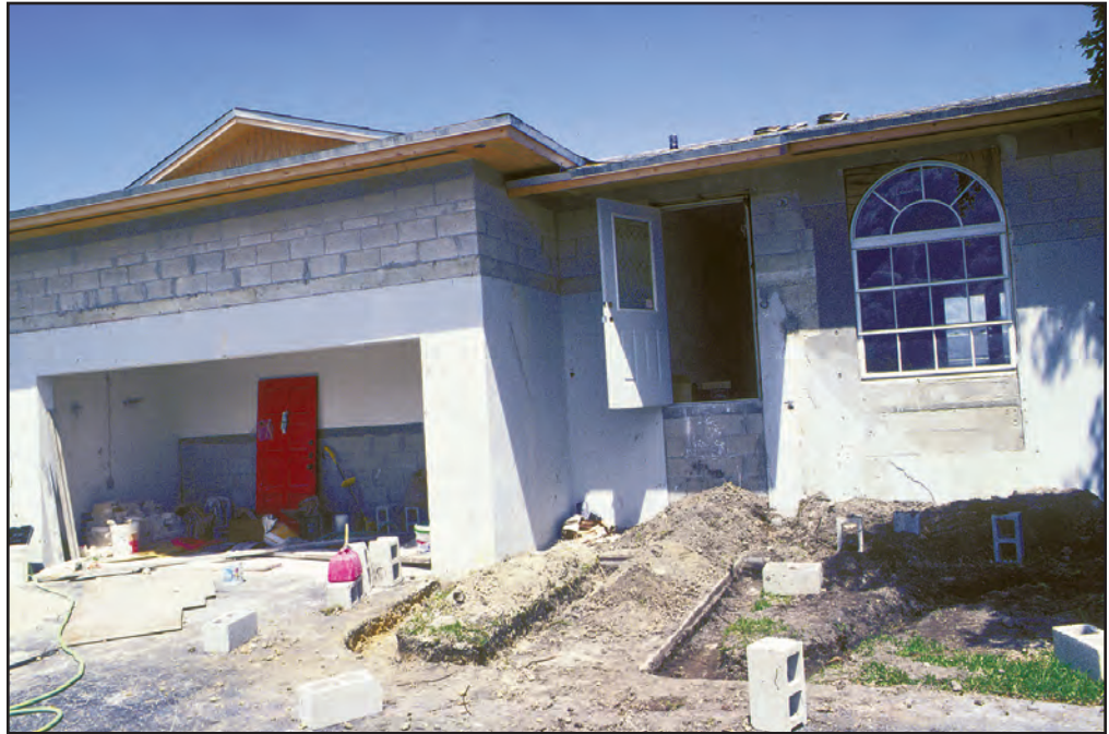
Figure 29 Windows and doors are added. The height of the raised front door shows the amount of elevation.
