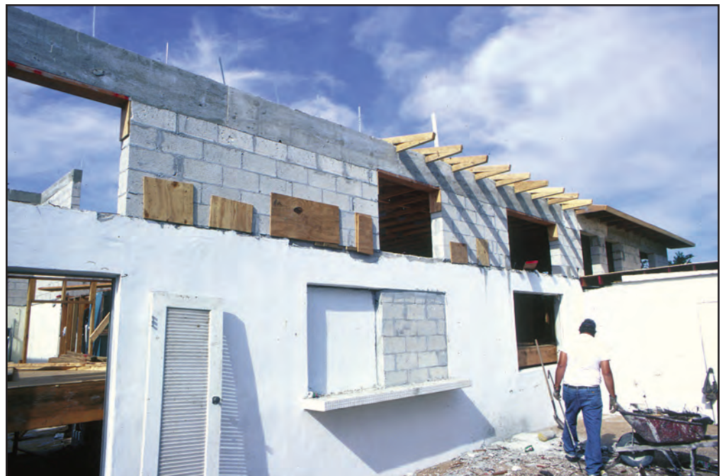
Figure 67 The extended first-story walls.
