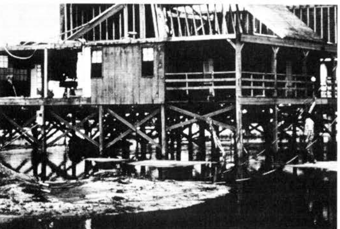
Figure 4.23. Diagonal Bracing
