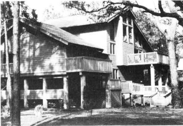
Figure 4.3. Elevation by Posts
