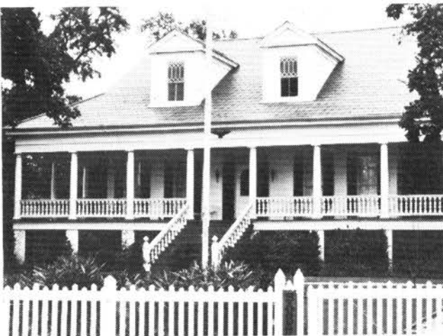
Figure 4.15. Pier Foundations
