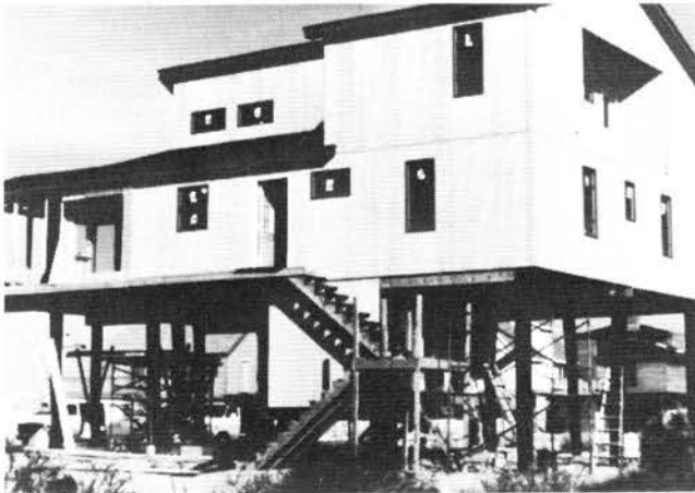
Figure 4.14. Pile Foundations
