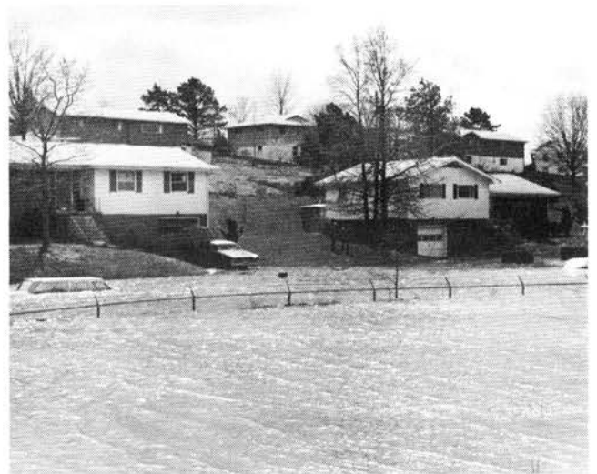
Figure 2.7. Improperly Sited Streets Can Block Emergency Egress and Access
