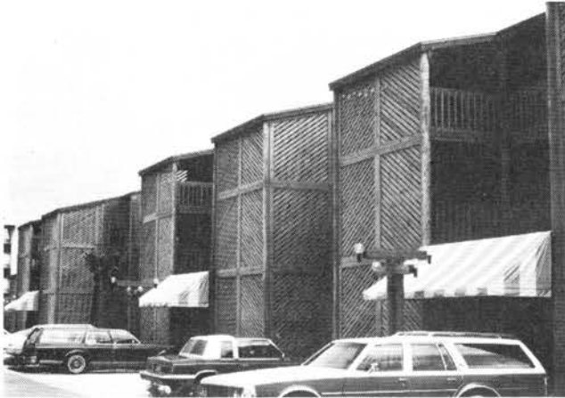
Figure 3.32. The diagonal battens used to enclose the stairwells for protection provide an aesthetically appealing screen-textural affect. The colored awnings also add a necessary highlight to an otherwise colorless exterior. Notice also the pole light fixture.
